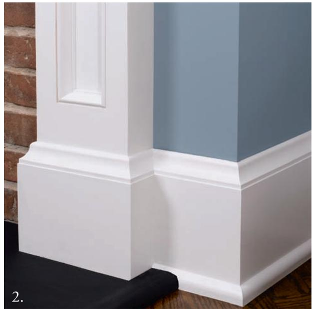
1. The depth and clarity of the casing helps to define doors, windows and returns, elevating them again to a place of prominence in the home. 2. The base molding wraps around the room aligning with the base on the mantel.
