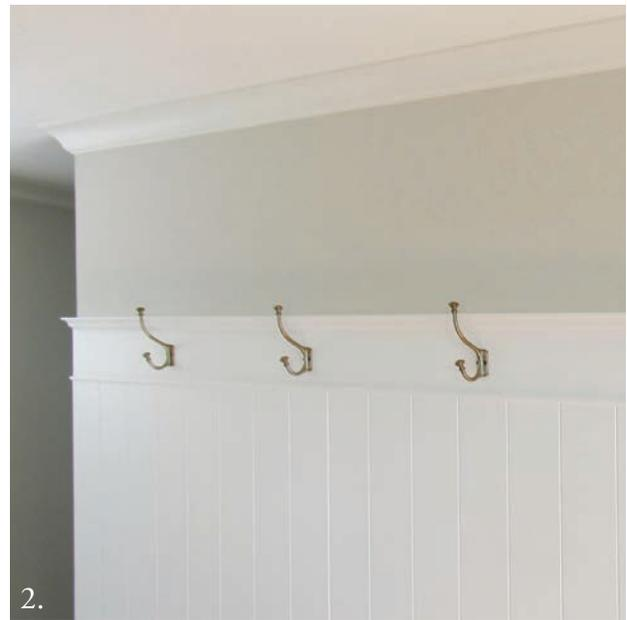
1. Craftsman header cap and window sill buildup connected by casing. 2. Example of the header buildup used to cap wainscot (shown with WindsorONE T&G profile WOTG wainscoting).
